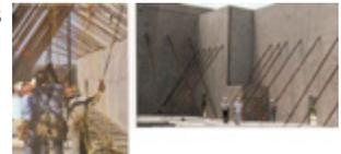
**Left: To properly stiffen the main bracing system, knee bracing should be attached to the main brace, at or very near the main brace's mid-point, creating a 90-degree angle with the main brace. Above: At a corner, the bracing must be intertwined to maintain support for the panels.**
