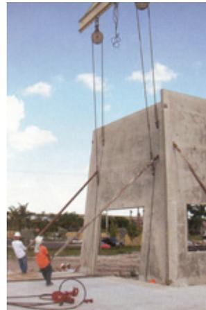
**Braces are usually designed by the tilt-up hardware suppliers using their brace capacities for the various lengths required and wind loadings. A safety factor of 1.5 is typical. Also, it is crucial to use hardware that matches the braces selected for the project. Improper matching may lead to fatigue or movement of the panels during this critical stage. The**
