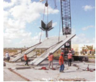
**After a panel has been set, but before the crane releases it, temporary erection braces must be installed to hold the panel plumb and in position, and provide resistance from wind. The minimum requirement is two braces per panel, but with the larger panels common today, additional bracing may be needed.**
