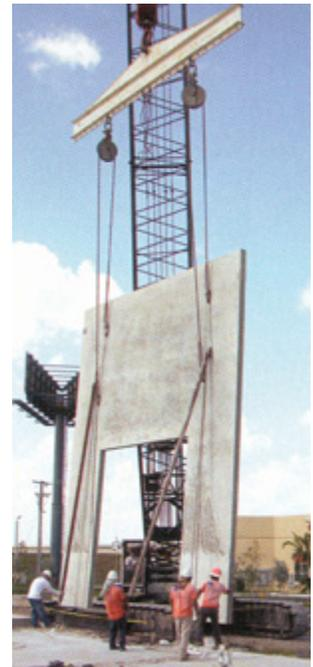
**Braces are usually made of steel pipe with approximately 18 inches of screw adjustment at the lower end. The upper end is bolted to an embedded wall brace insert, and the lower end attaches to the concrete slab, most often by a post-installed bolt.**
