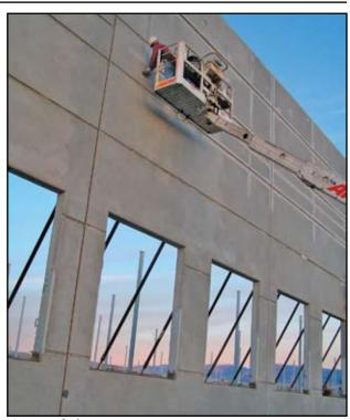
precast concrete systems. Inadvertently, these provisions are extending to site-cast tilt-up construction, because tilt-up falls under the broad umbrella of precast concrete. Although the precast concrete seismic provisions may at first seem awkward to apply to tilt-up construction, a rational approach can be developed by understanding the intent of the provisions.
