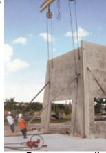
Braces are usually designed by the tilt-up hardware suppliers using their brace capacities for the various lengths required and wind loadings. A safety factor of 1.5 is typical. Also, it is crucial to use hardware that matches the braces selected for the project.Improper matching may lead to fatigue or movement of the panels during this critical stage. The
