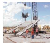
After a panel has been set, but before the crane releases it, temporary erection braces must be installed to hold the panel plumb and in position, and provide resistance from wind. The minimum requirement is two braces per panel, but with the larger panels common today. additional bracing may be needed.
